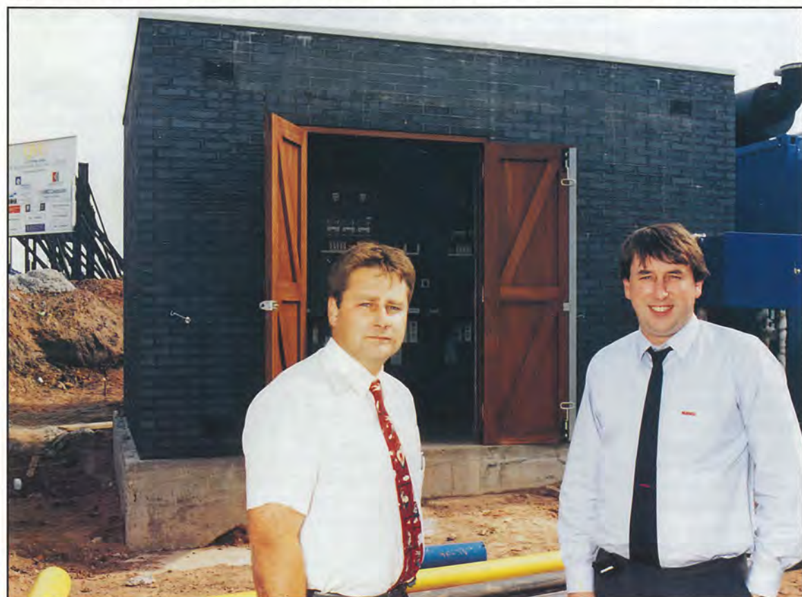
New connections form an important part of Merseyside Region's work. Engineer Jim Powell (left) and Foreman Andy Skarratts are pictured outside a new substation constructed to serve the QVC television shopping channel's call centre in Kirkby.
